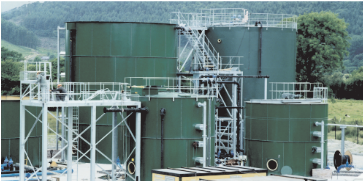
Project photographed during construction.
